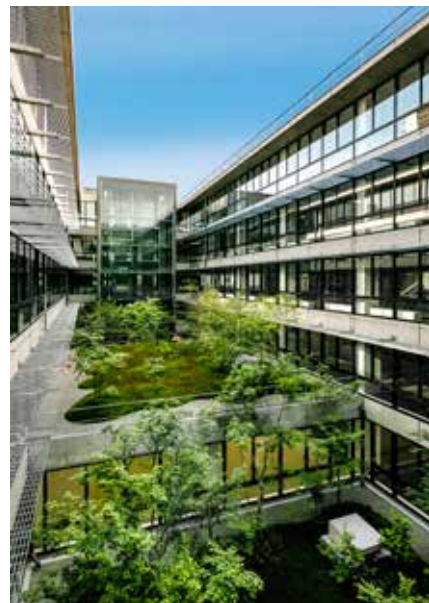
Kyoto City Hall Branch Office
