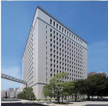
East Building of Nippon Life Insurance Company Head Office
