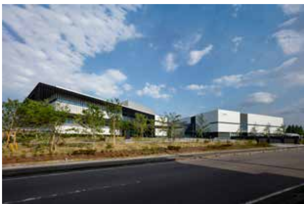
Takasago Thermal Engineering Innovation Center
